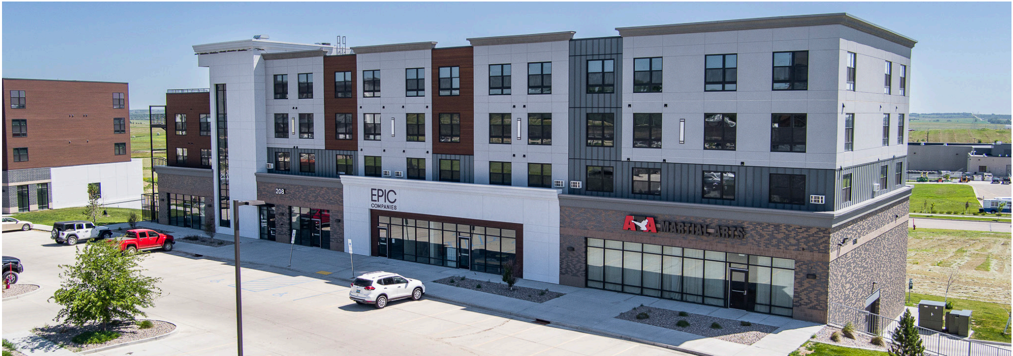
208 Building C - 1st Floor
